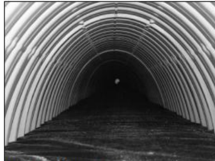
Looking down the Isolator Row
