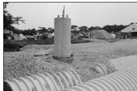
Figure 15 – Chamber bed placed around light post.
